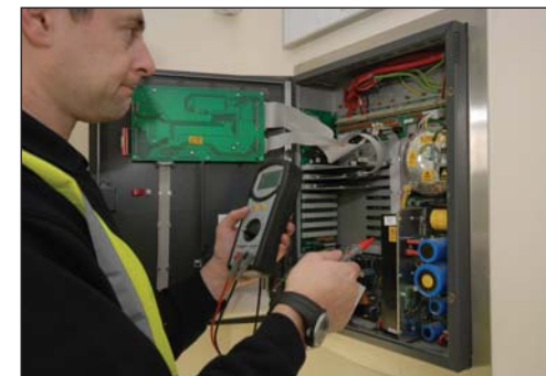
Fig 9 - Testing of Wiring
