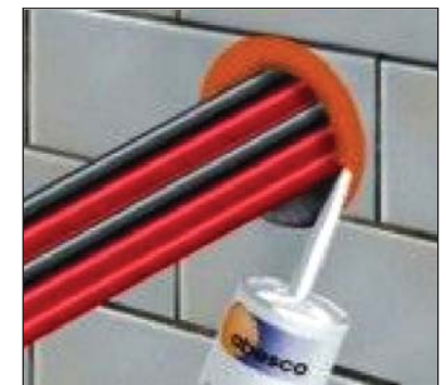
Fig 7 - Fire sealing of holes using a fire rated mastic
